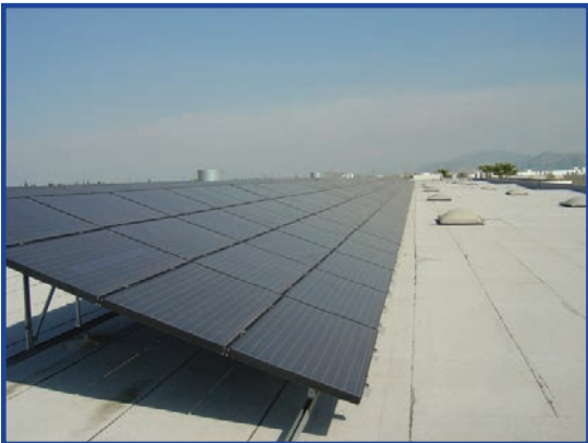
A 250 kilowatt solar photovoltaic system on the roof of a Majestic warehouse in Ontario, CA. This system eliminates 25% of the occupant's electricity bill.
