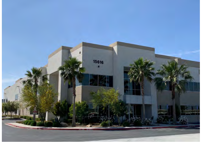
Southeast Corner View
