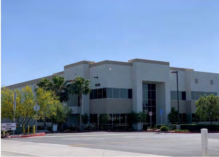
Northeast Corner View
